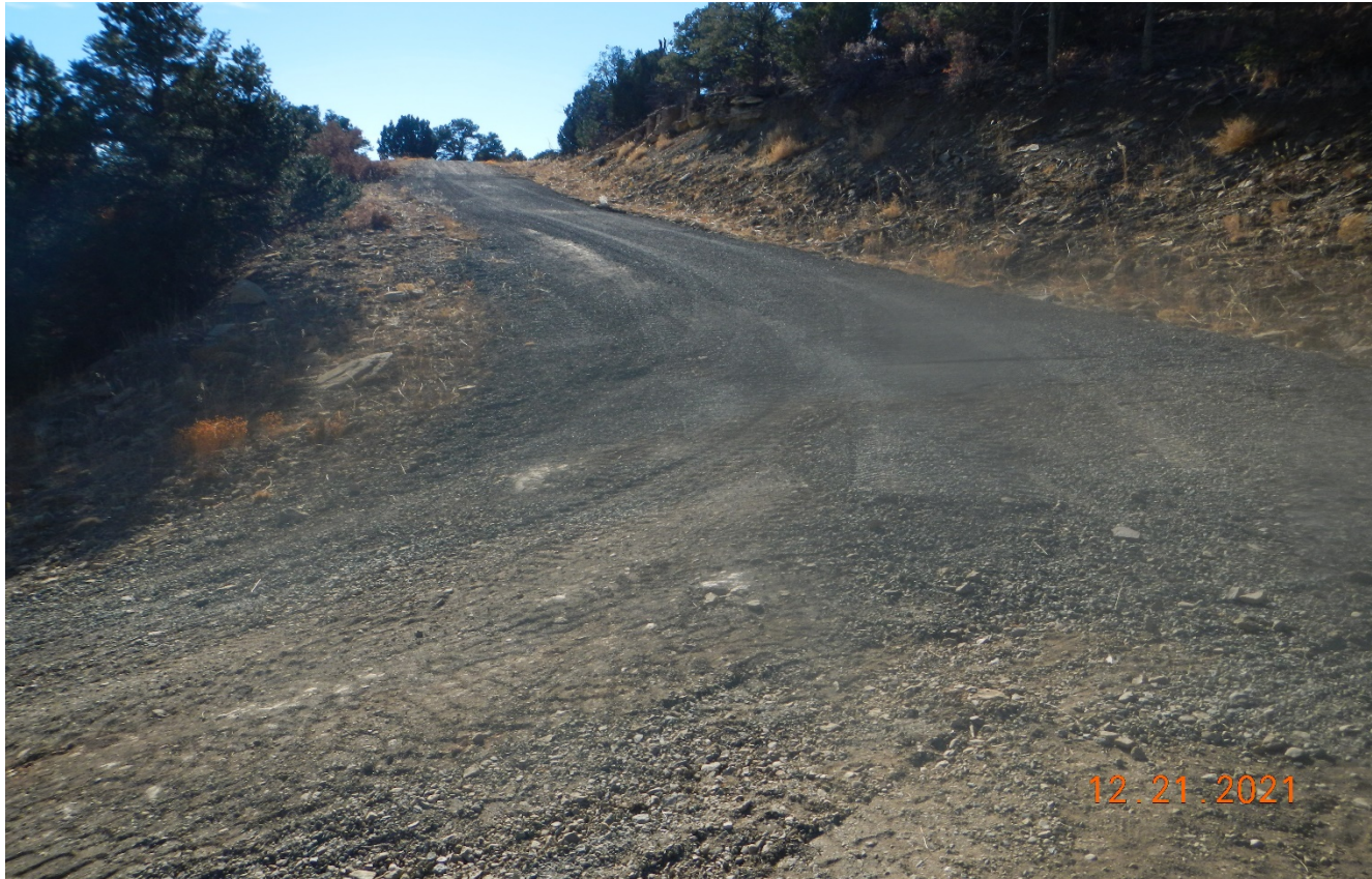
Photo 2. The area of erosion along the switch back of the road has been repaired.
