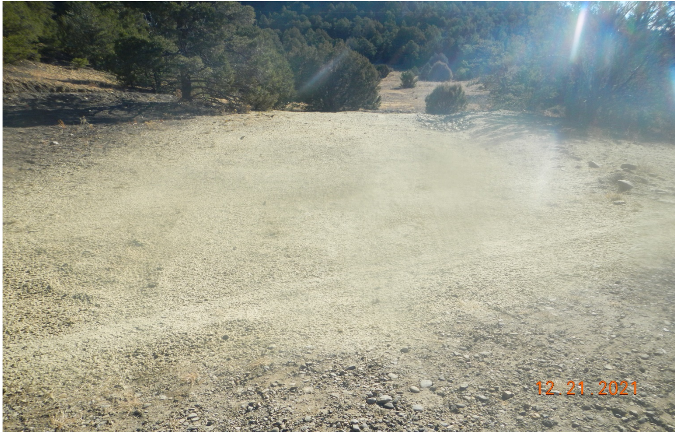
Photo 2. Facing toward the southeast side of the location. This area has been seeded and stabilized with hydro-mulch.
