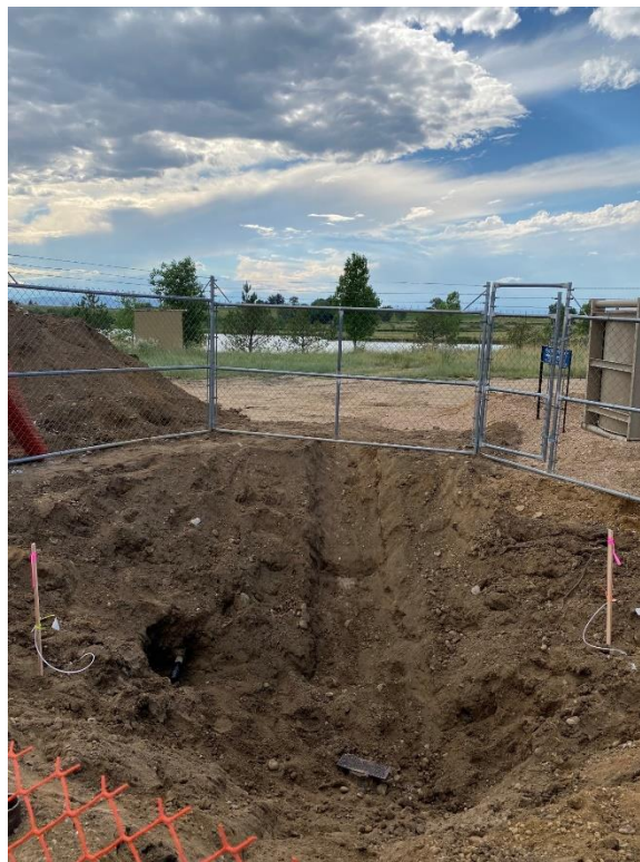
Williams 18-29 – Wellhead Excavation
