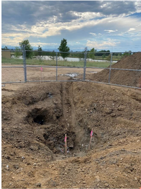
Williams 36-30 – Wellhead Excavation
