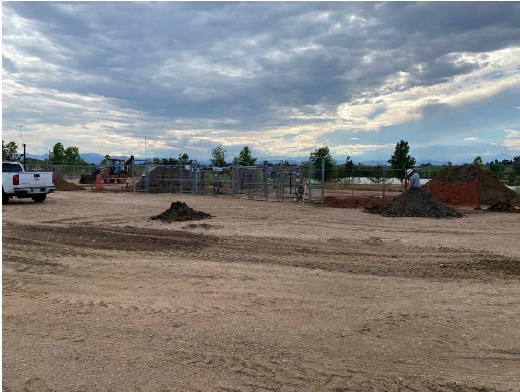
Williams 18-29 and 36-20 – Wellheads Excavation
