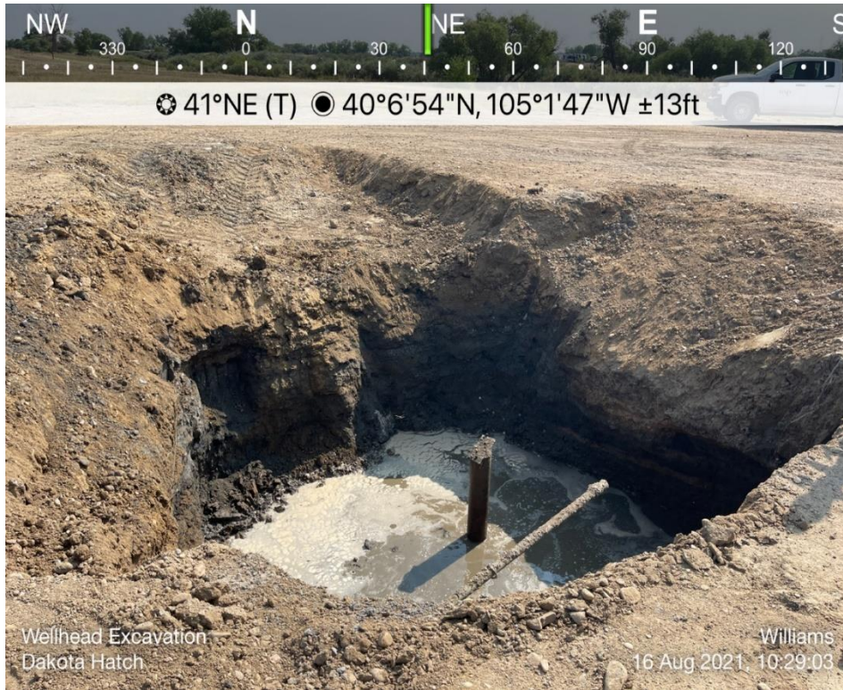
Williams 36-20 – Wellhead Excavation
