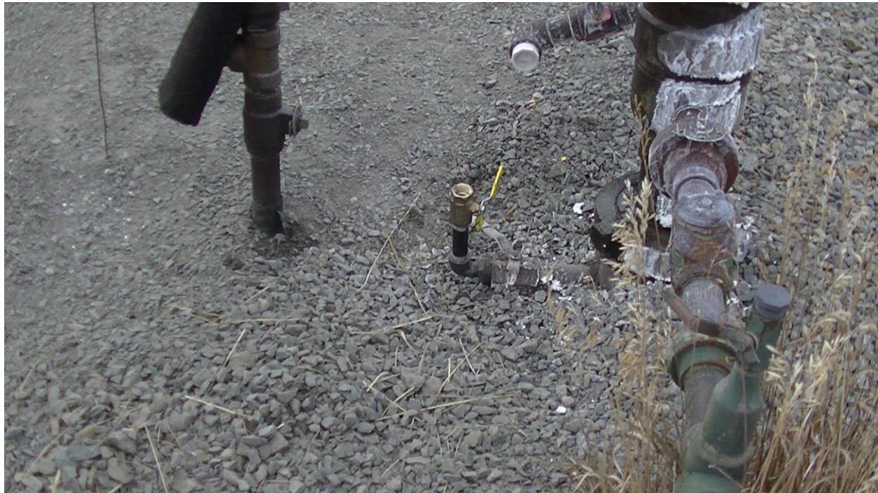
Installed appropriate fittings to allow bradenhead visual inspection as per Rule 419.a
