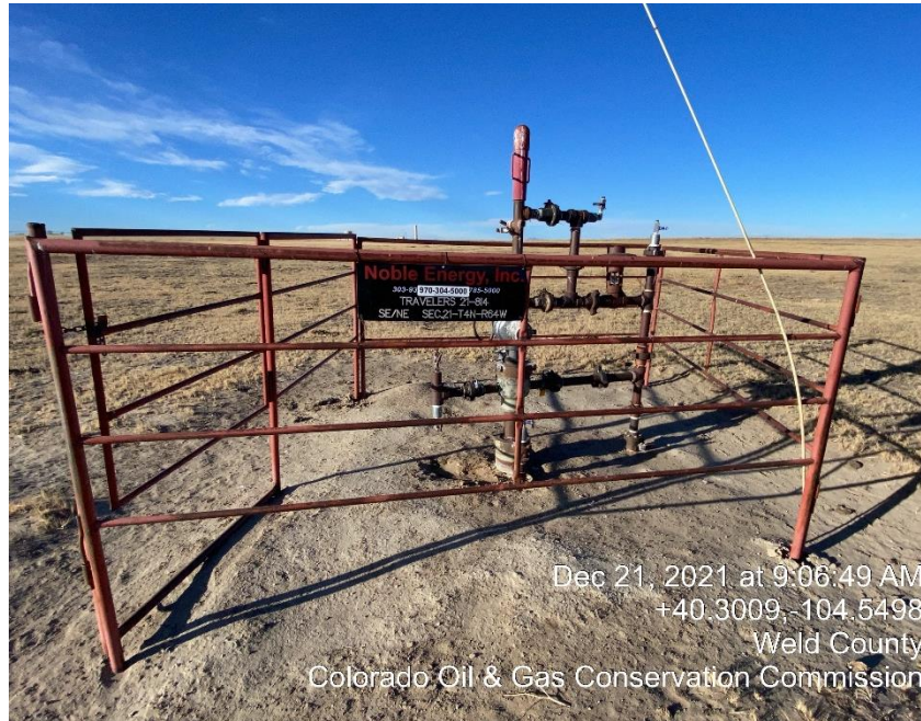
Well & Removed Unused Equipment
