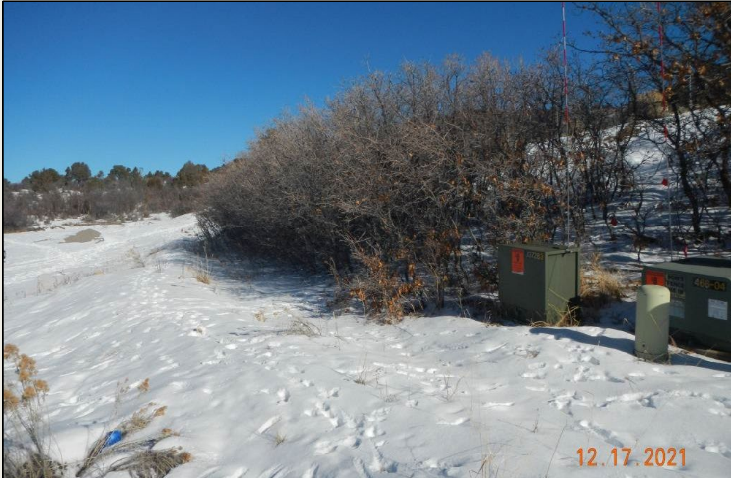
Photo 3. View of the western project area from the southwestern corner facing northward. Berm is in place along southern edge of the project area.
