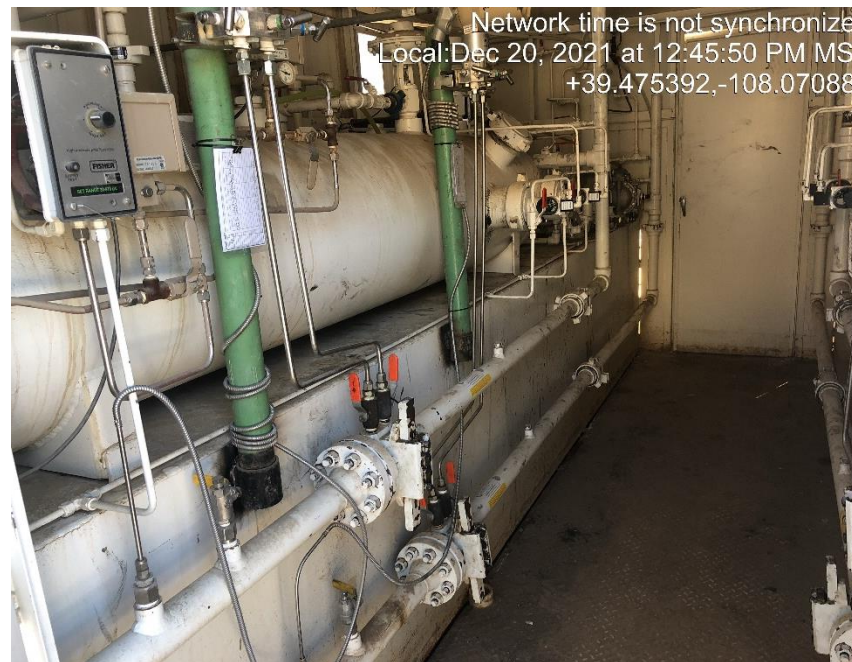
Photo #5443 Storage tank located under the horizontal separator.
