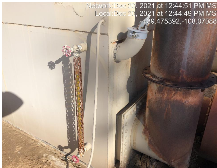
Photo #5442 Sight glass indicates the storage tank is full of an unknown fluid.
