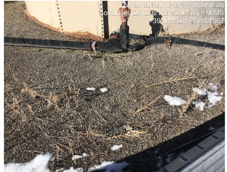
Photo #5445 Debris inside tank containment.
