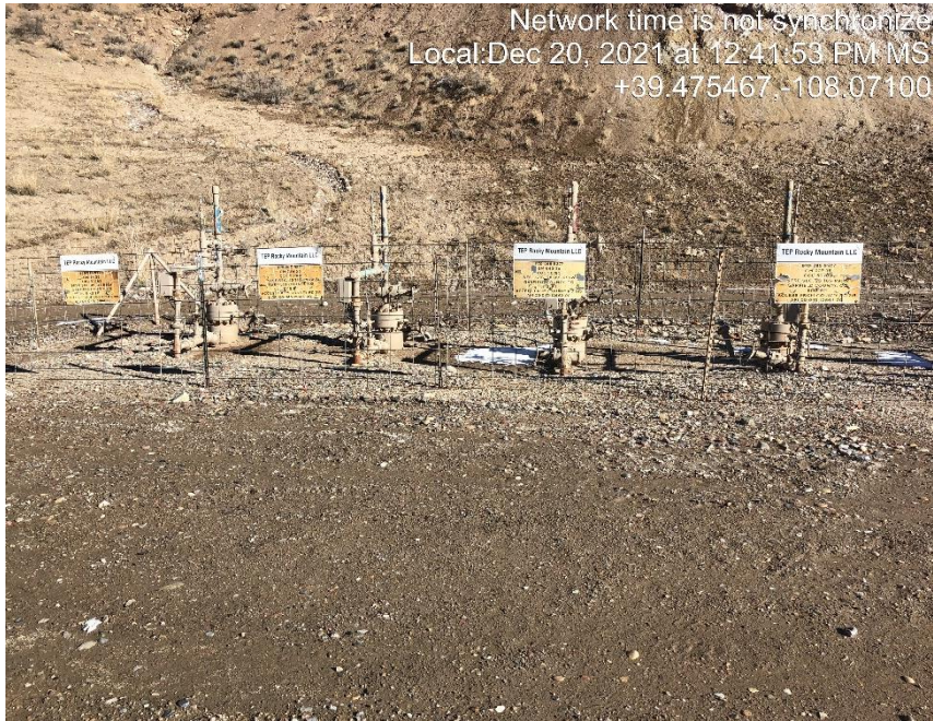
Photo #5440 Multiple wellhead signs weathered and not legible.
