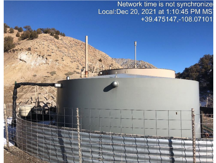
Photo #5446 Vent pipe open ended and venting. No PRV or bull plug on vent pipe.
