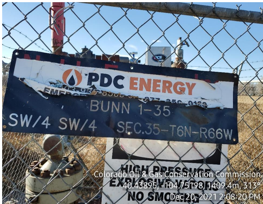
Photo 1: Wellhead Sign; emergency # not legible
