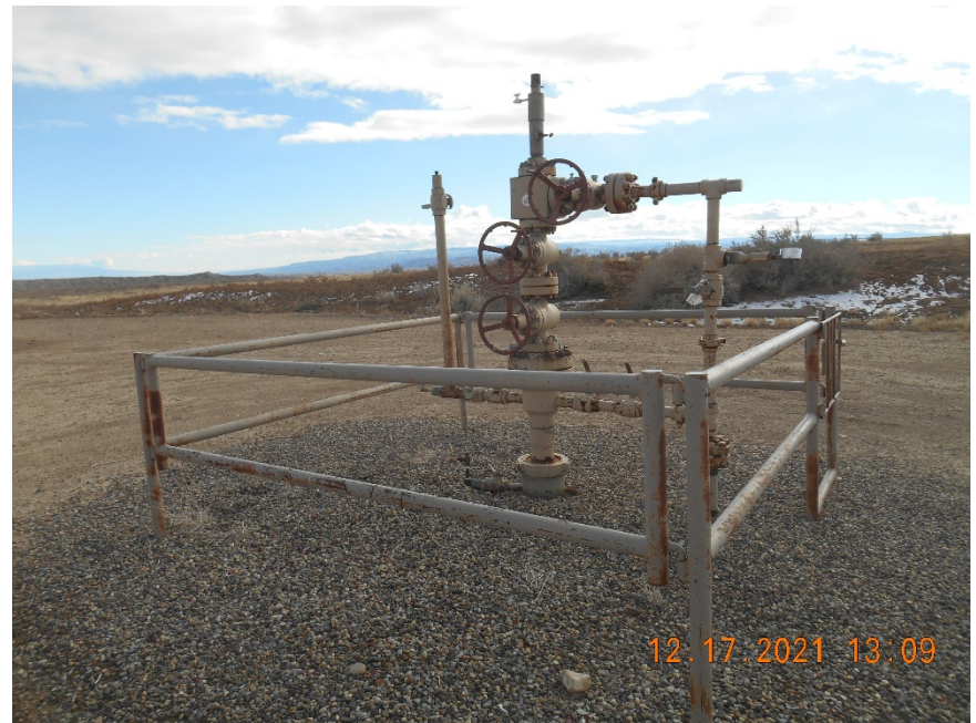
Wellhead Temporarily Abandoned
