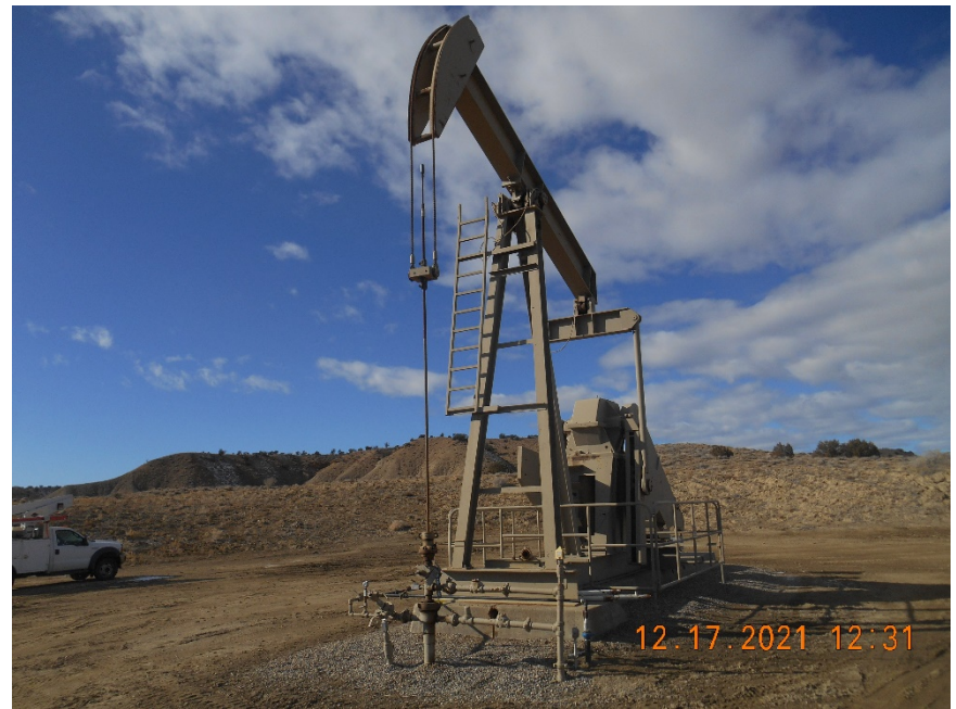
Wellhead with pump jack
