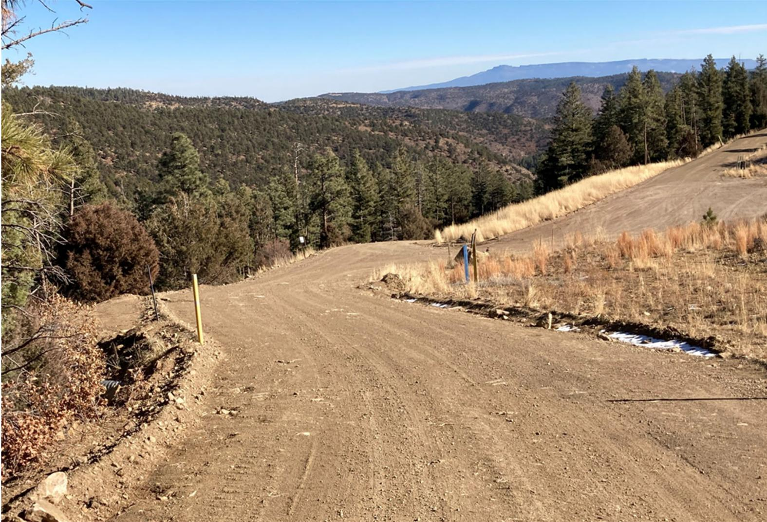
THE MAIN LEASE ROAD SURFACE WAS REGRADED AND CROWNED. THIS CONFIGURATION WILL CREATE SHEET FLOW AND ELIMINATE THE TIRE RUTS/SURFACE EROSION. THE ROAD SURFACE WAS COMPACTED BY UTILIZING A VIBRATION SOIL COMPACTION ROLLER TO PROVIDE STABILIZATION.
