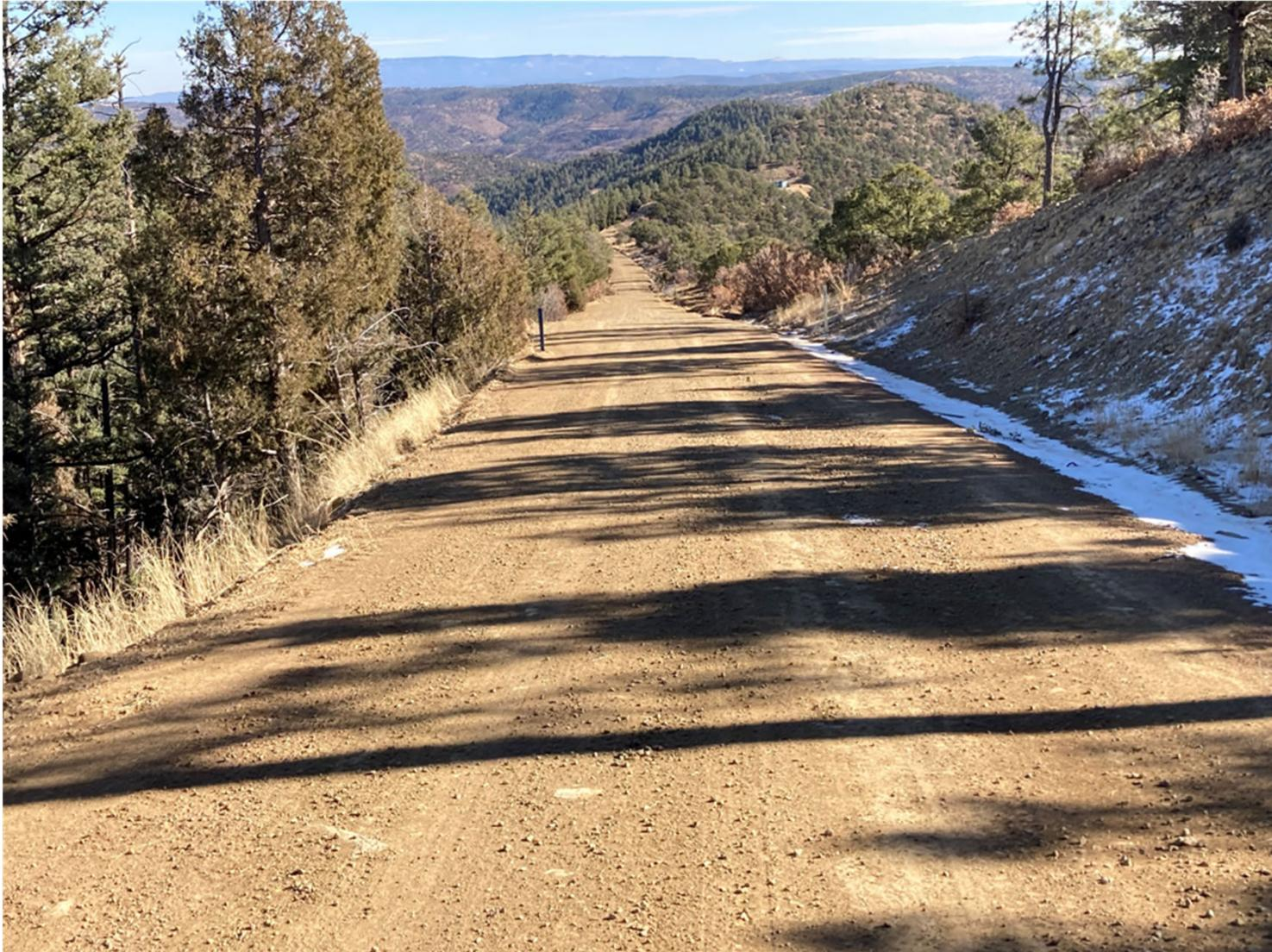
THE MAIN LEASE ROAD SURFACE WAS REGRADED AND CROWNED. THIS CONFIGURATION WILL CREATE SHEET FLOW AND ELIMINATE THE TIRE RUTS/SURFACE EROSION. THE ROAD SURFACE WAS COMPACTED BY UTILIZING A VIBRATION SOIL COMPACTION ROLLER TO PROVIDE STABILIZATION.
