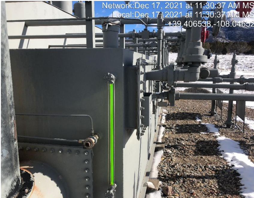
Photo #5410 Sight glass indicates the storage tank is full of an unknown fluid.
