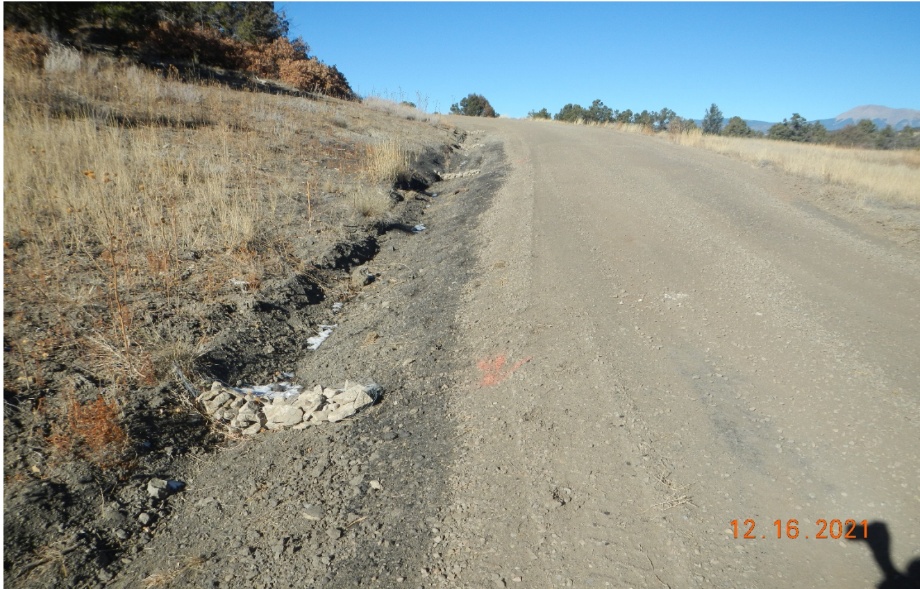
Photo 1. Facing northwest along the main access road. There are rock check dams installed along the side of the road.
