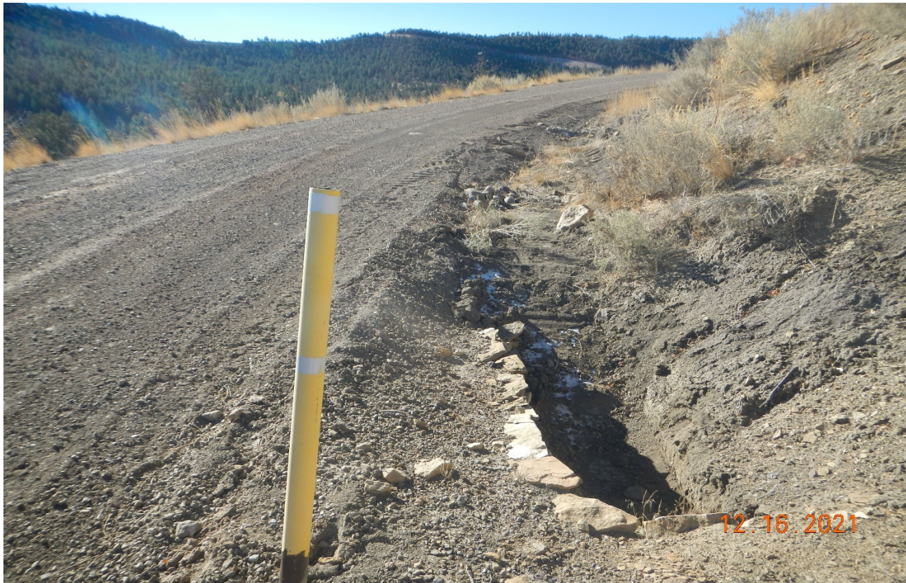
Photo 2. The culverts have been cleaned out and areas of erosion were repaired.
