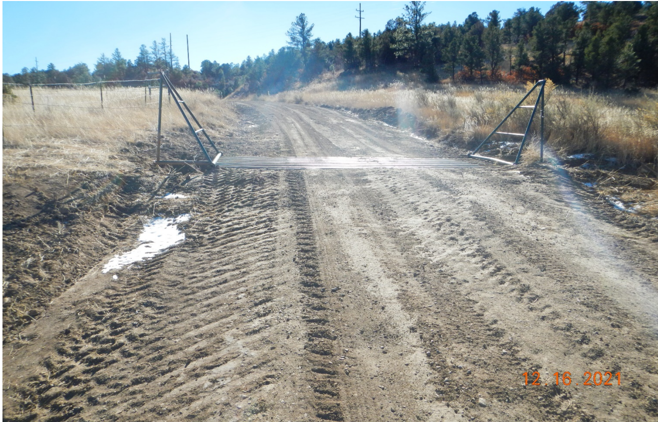
Photo 1. Facing southeast along the main access road. The access road has been regraded and sediment was cleaned out the cattle guard.
