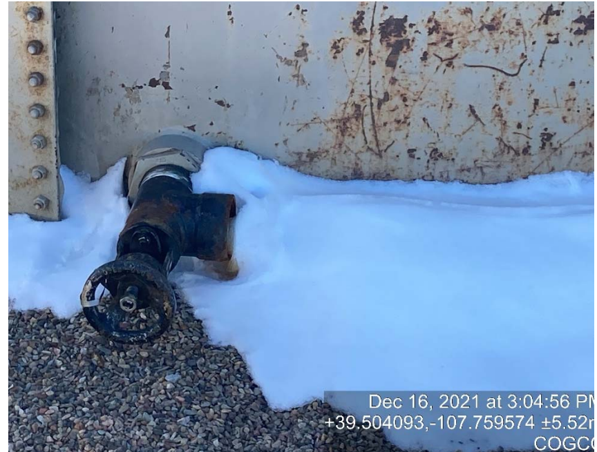
Load line lacking bull plug/cap
