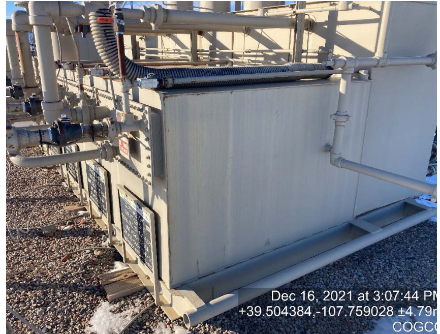
Storage tank lacking labeling
