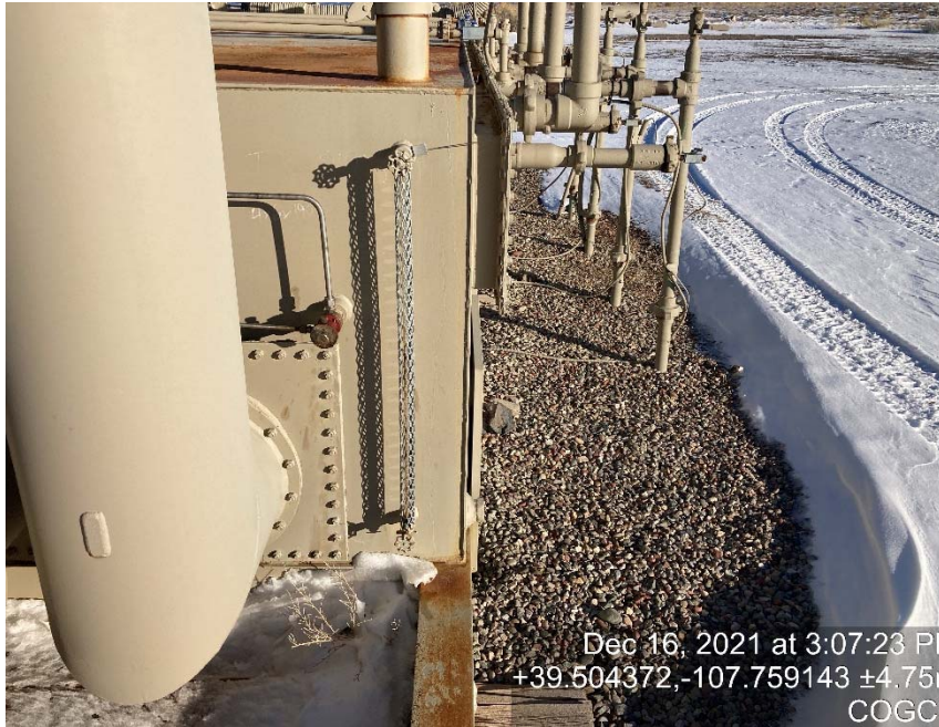
Storage tank lacking labeling/sight glass shows fluid
