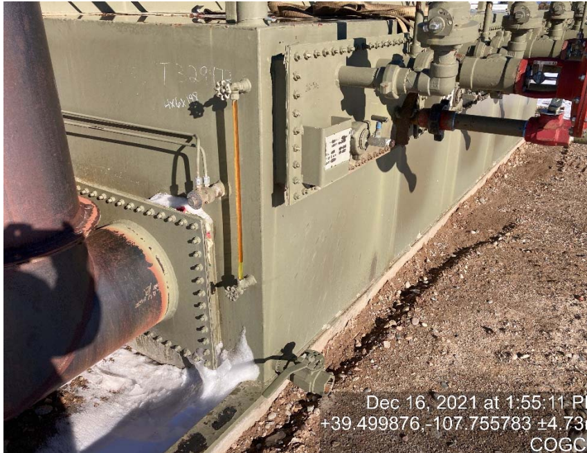
Storage tank lacking labeling/sight glass shows fluid
