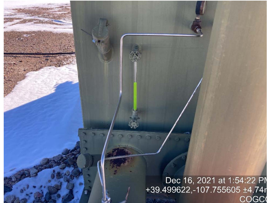
Storage tank lacking labeling/sight glass shows fluid
