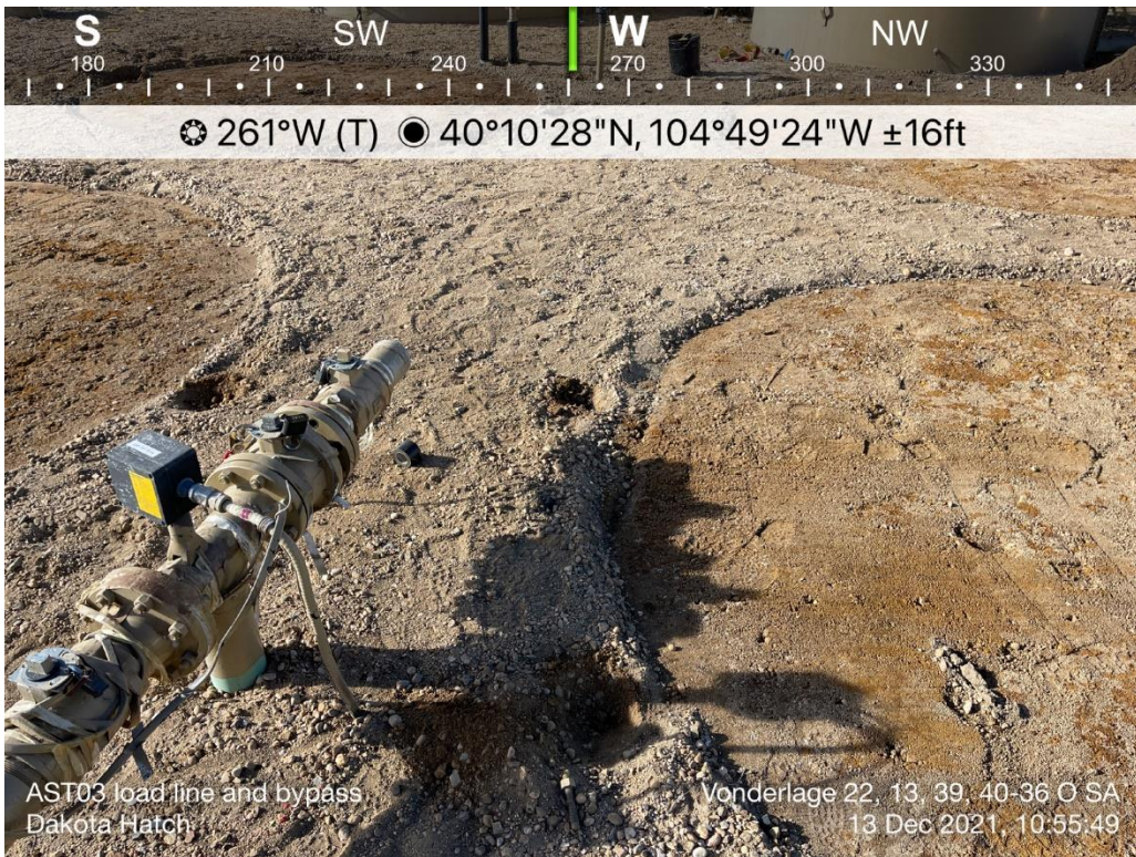
Above ground storage tank 03 (AST03) – Load line and bypass
