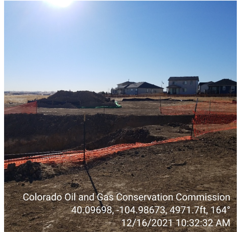
Photo 2 – Excavation. Fencing down. Silt fence damaged by wind.
