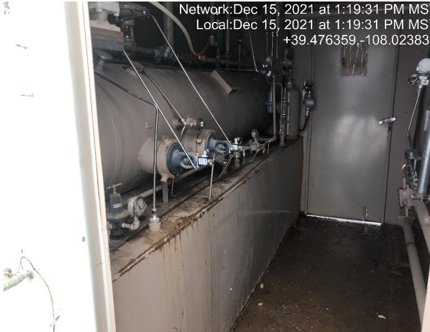
Photo #5402 Storage tank located under the horizontal separator.
