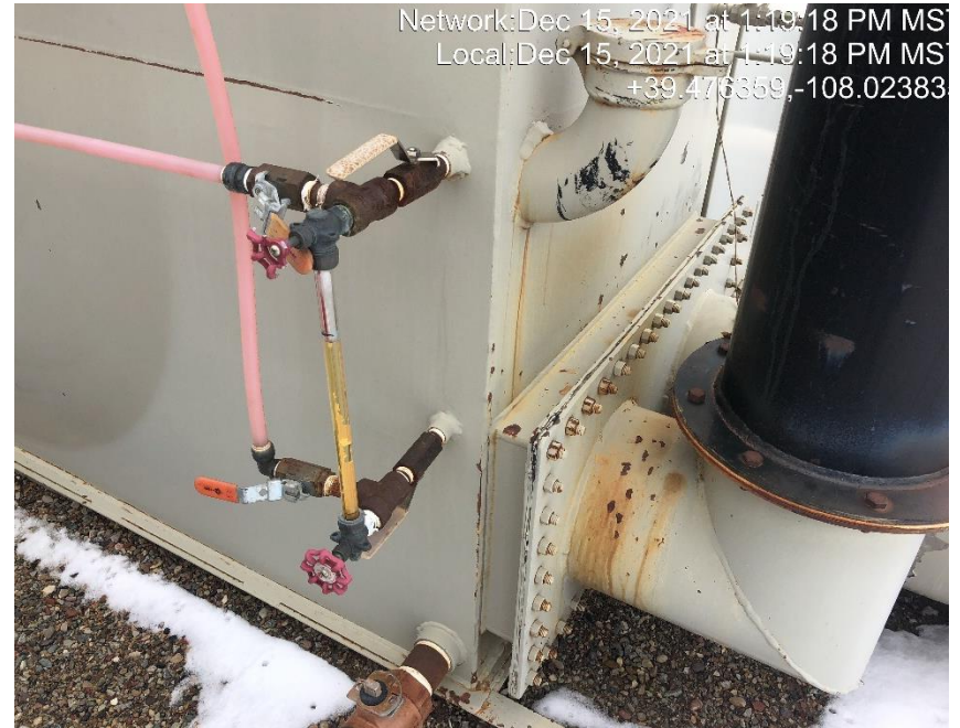
Photo #5401 Sight glass indicates the storage tank is full of an unknown fluid.
