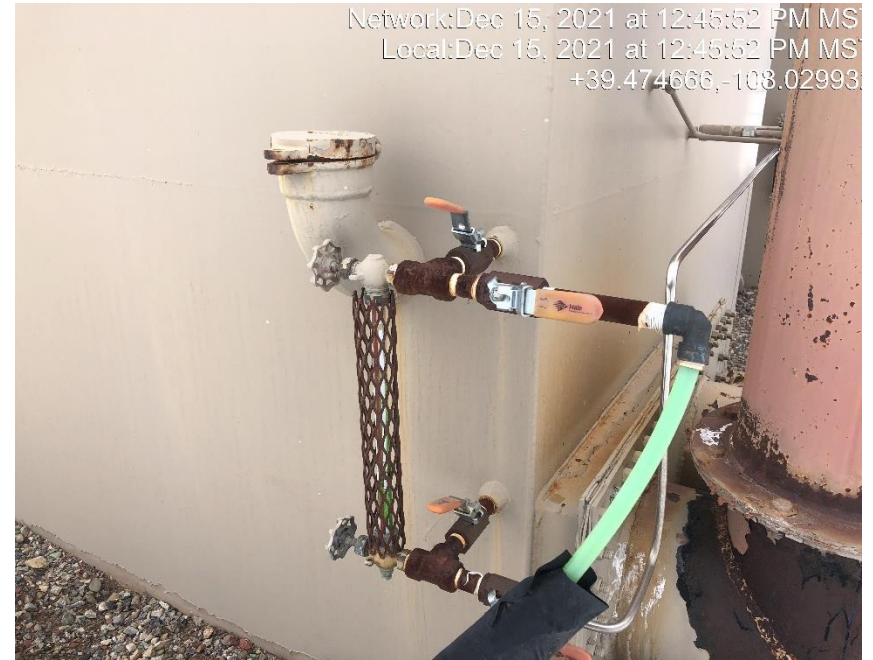
Photo #5396 Sight glass indicates the storage tank is full of an unknown fluid.
