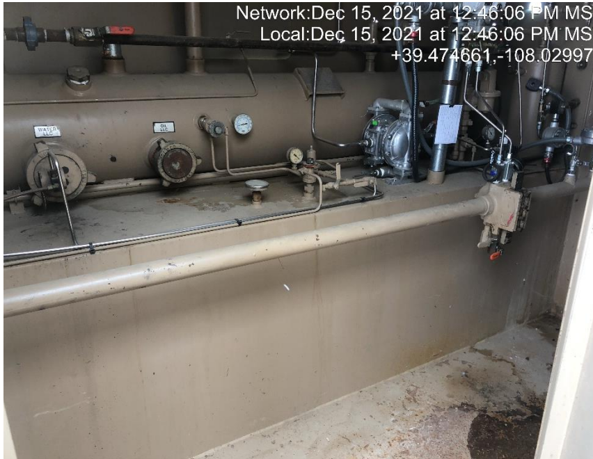
Photo #5397 Storage tank located under horizontal separator.
