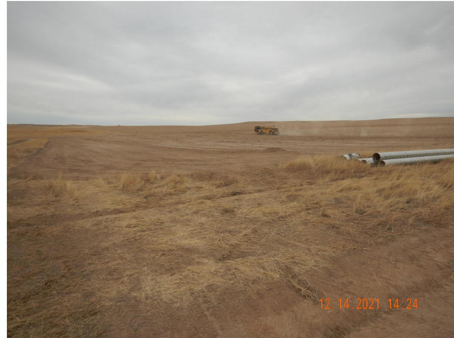
Photo 2. Photo taken from the southwestern location, facing North. Photo illustrates topsoil salvage operations are underway.
