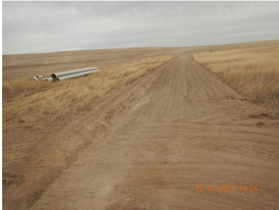
Photo 1. Photo taken from the southwestern location, facing East. Photo illustrates a ditch and berm BMP which has been installed around the entire perimeter of location.
