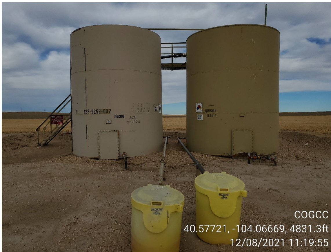
Photo 2: Crude Oil and Produced Water AST
