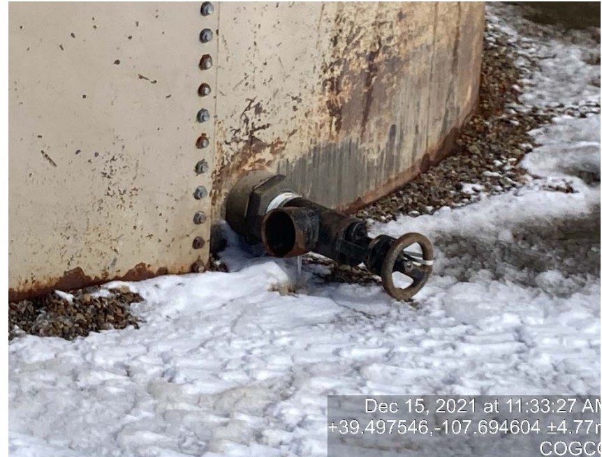
Load line lacking bull plug/cap
