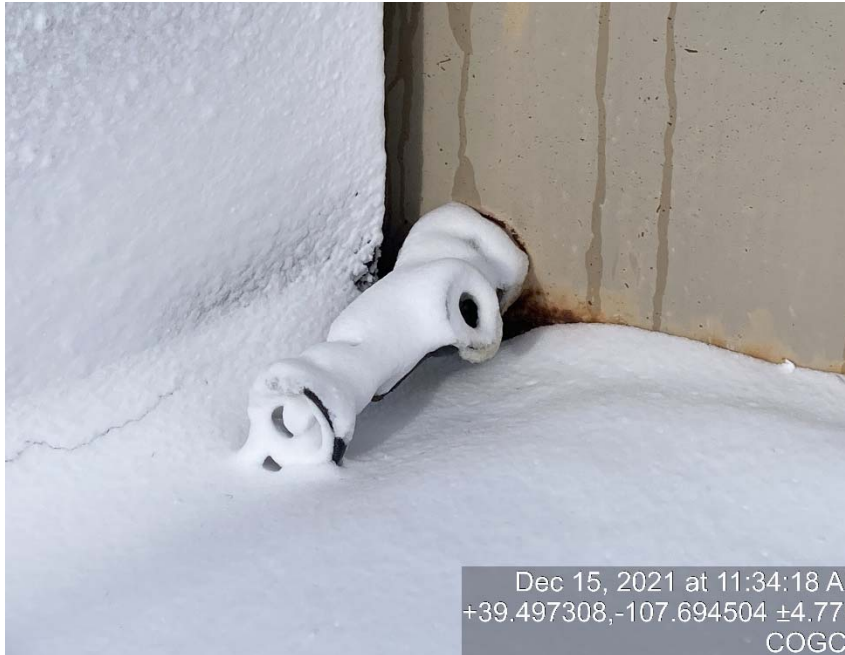
Load line lacking bull plug/cap
