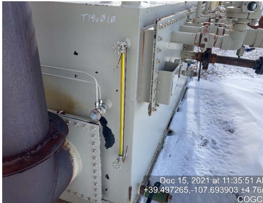
Sight glass shows fluid in storage tank
