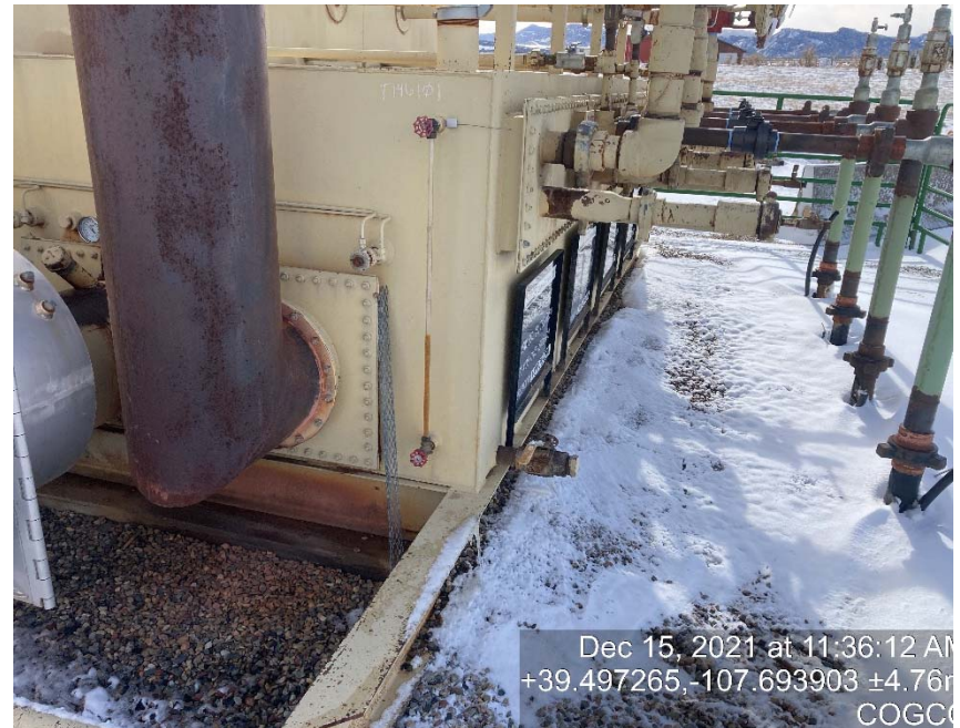
Sight glass shows fluid in storage tank
