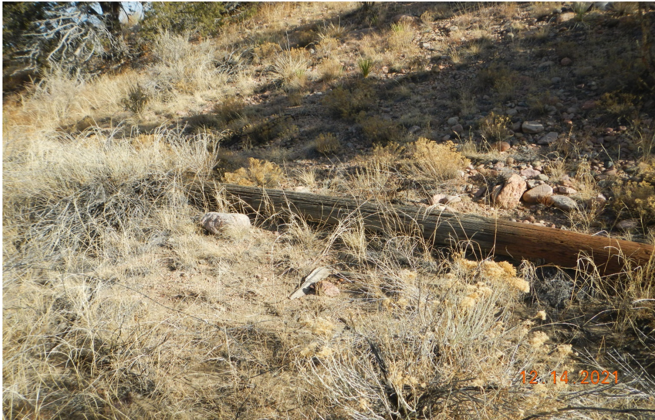
Photo 2. There is an abandoned powerpole that remains which needs to be removed.
