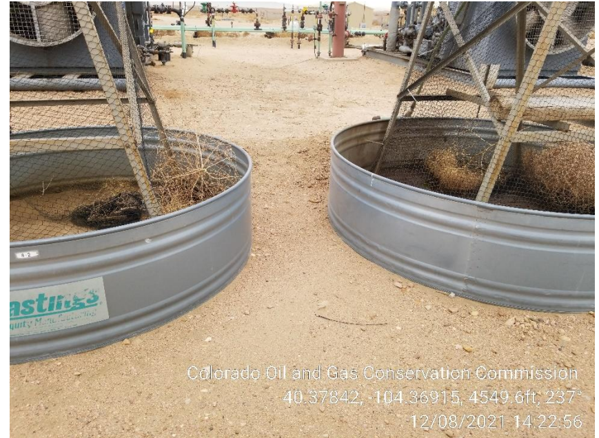
Photo 6 – Day Tank – Netting Inadequate
