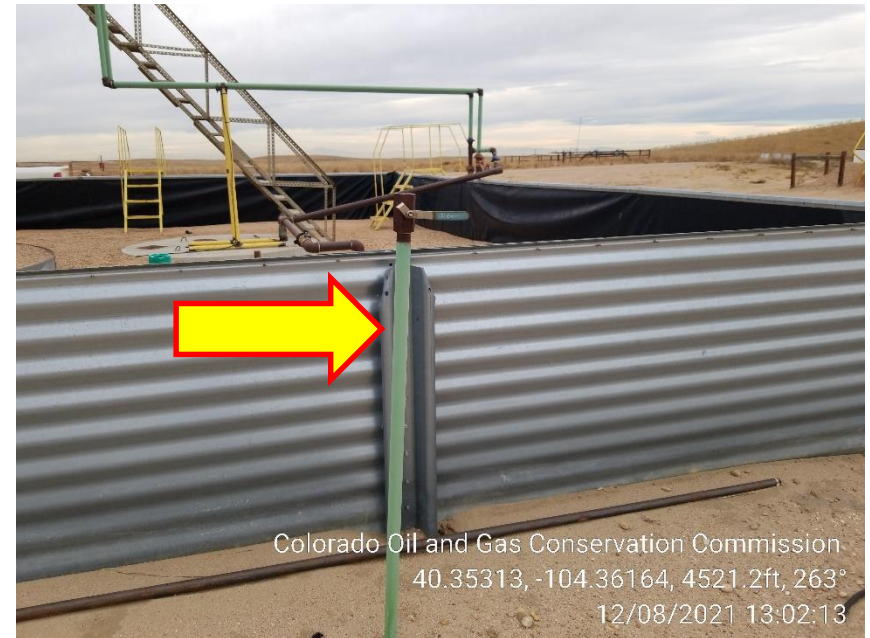
Photo 6 – Unmarked Riser
