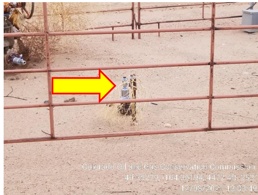
Photo 8 – Unmarked Risers
