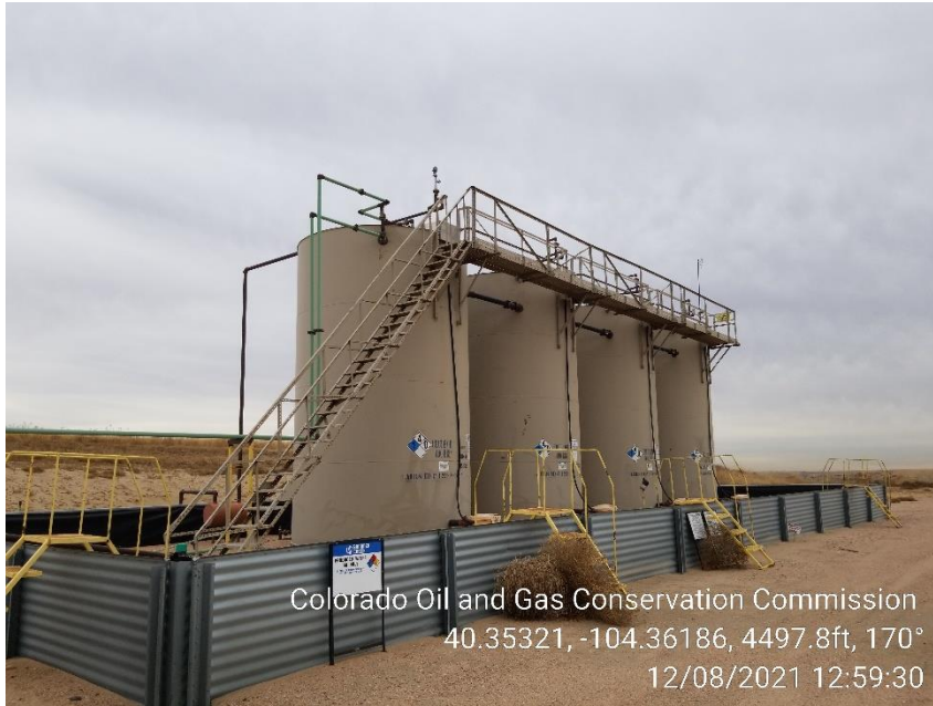
Photo 3 – Tank Battery
