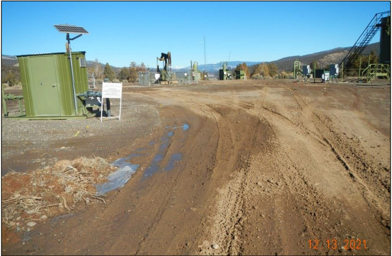
Photo 1. View of the project area from the northwestern corner facing center.
