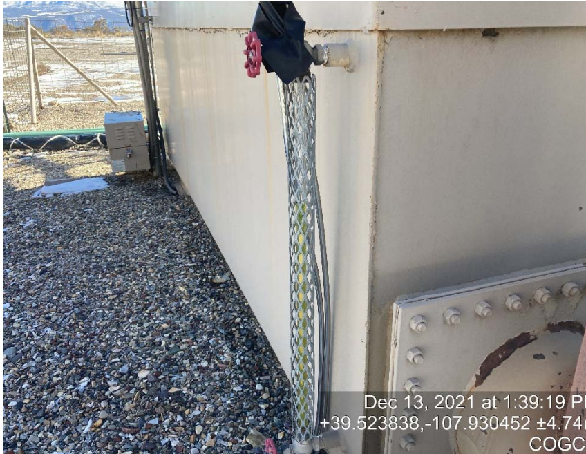
Sight glass shows fluid in storage tank
