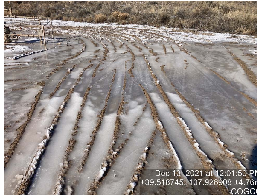
Lack of stabilization/compaction
