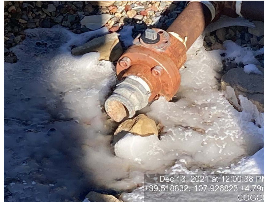
Load lines lacking caps/bull plugs
