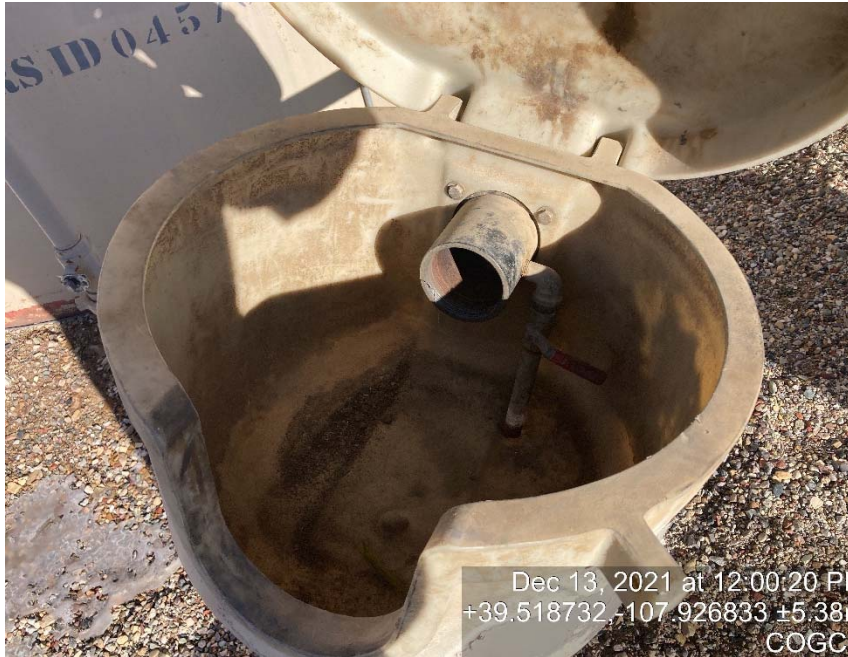
Load lines lacking caps/bull plugs
