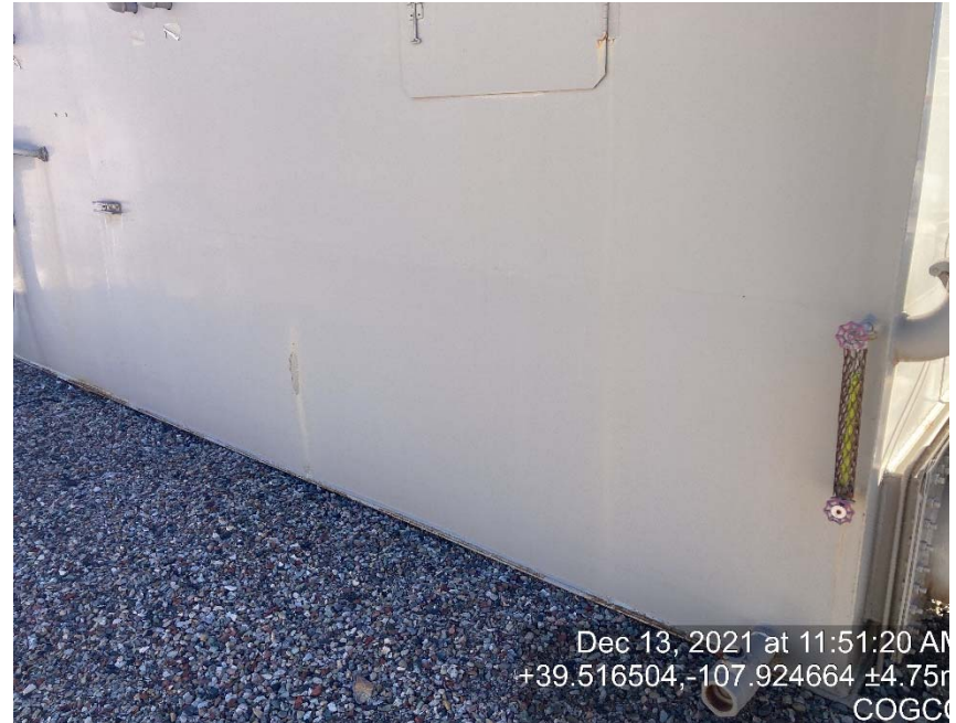
Sight glass shows fluid in storage tank
