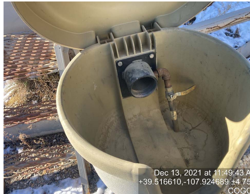
Load lines missing caps/bull plugs
