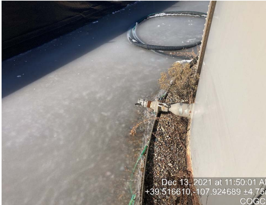
Load lines missing caps/bull plugs
