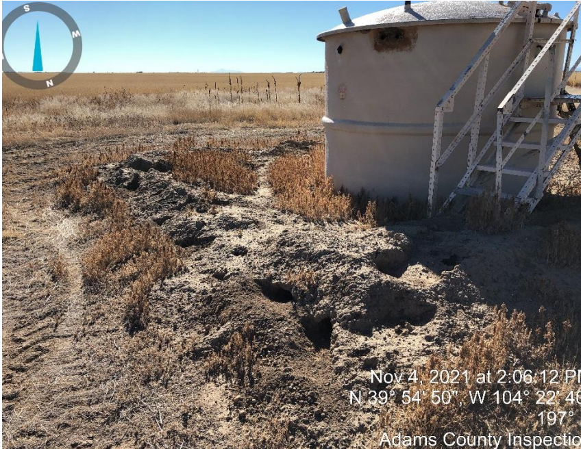
Photo #5 Unmaintained berm
