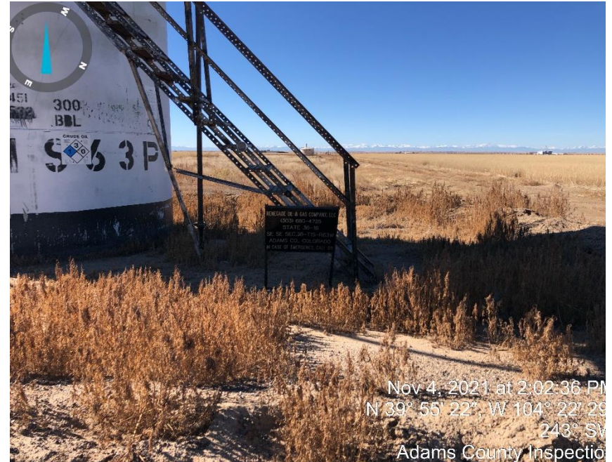
Photo #6 unmaintained berm.
