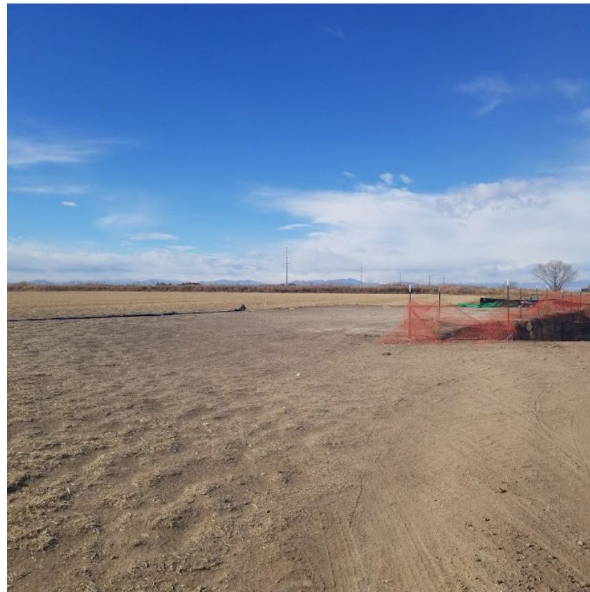
Photo 4 – Site overview; silt fence damaged by wind.
