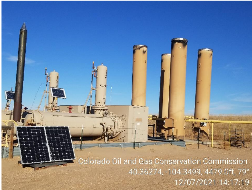
Photo 7 – Separators and ECDs
