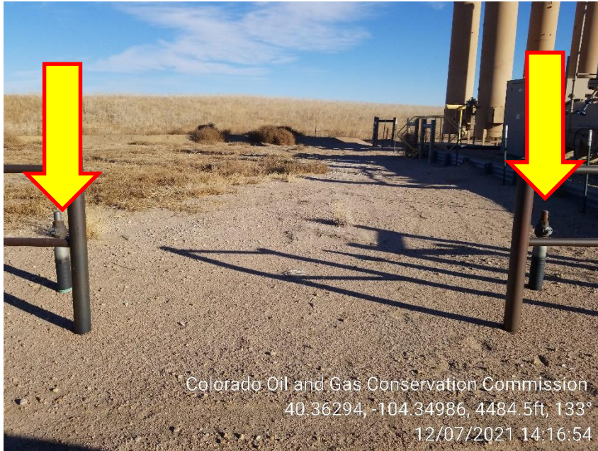
Photo 5 – Unmarked Risers
