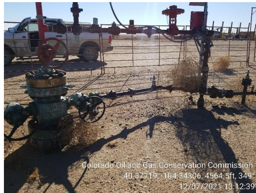
Photo 4 – Second Wellhead from the West missing Wellhead Sign
