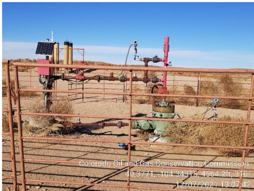
Photo 3 – Second Wellhead from the West missing Wellhead Sign
