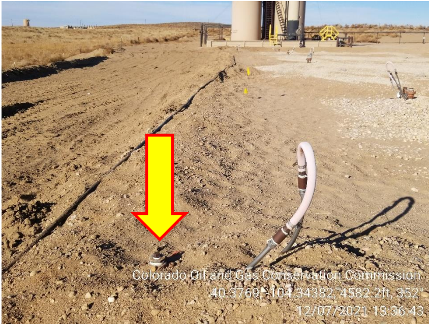
Photo 9 – Unmarked Riser
