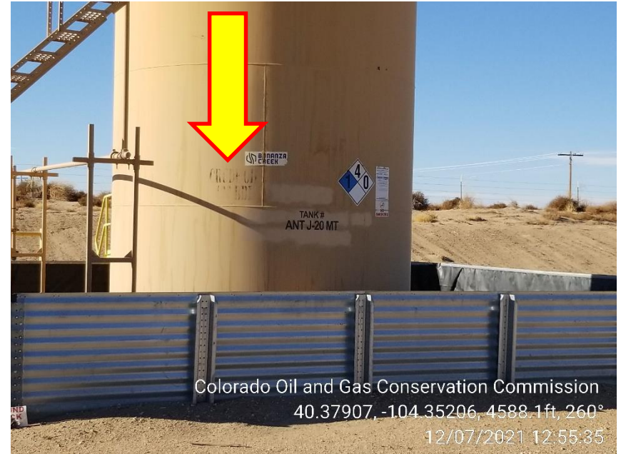
Photo 4 – Tank Battery – Content and Capacity Labels
