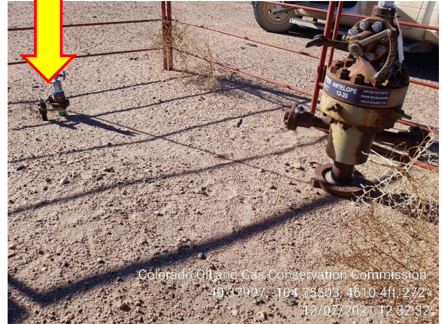
Photo 2 – 13-20 Wellhead – Unmarked Risers
