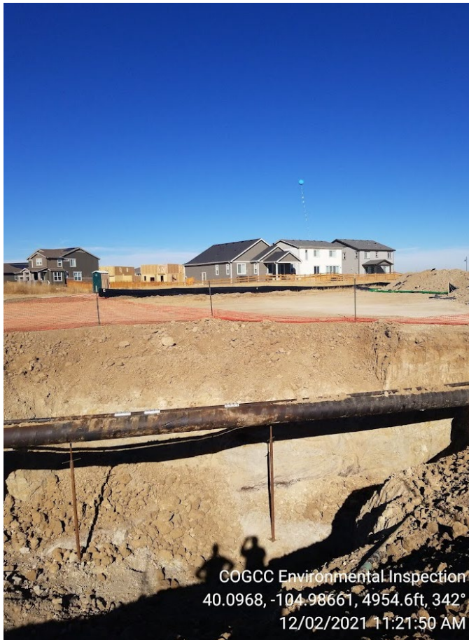
Photo 5 – 12/2/2021: Foreground: Remedial excavation and downed fencing. Background: Additional soils stockpiles.
