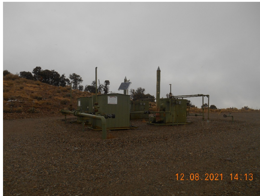
Separators and meter housings
