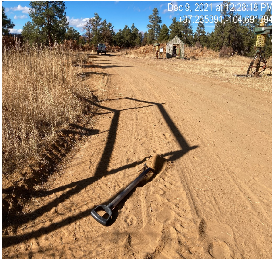
Photo 10. Facing north along the access road at the well site. The shovel placed in the road surface shows loose soils and lack of stabilization
