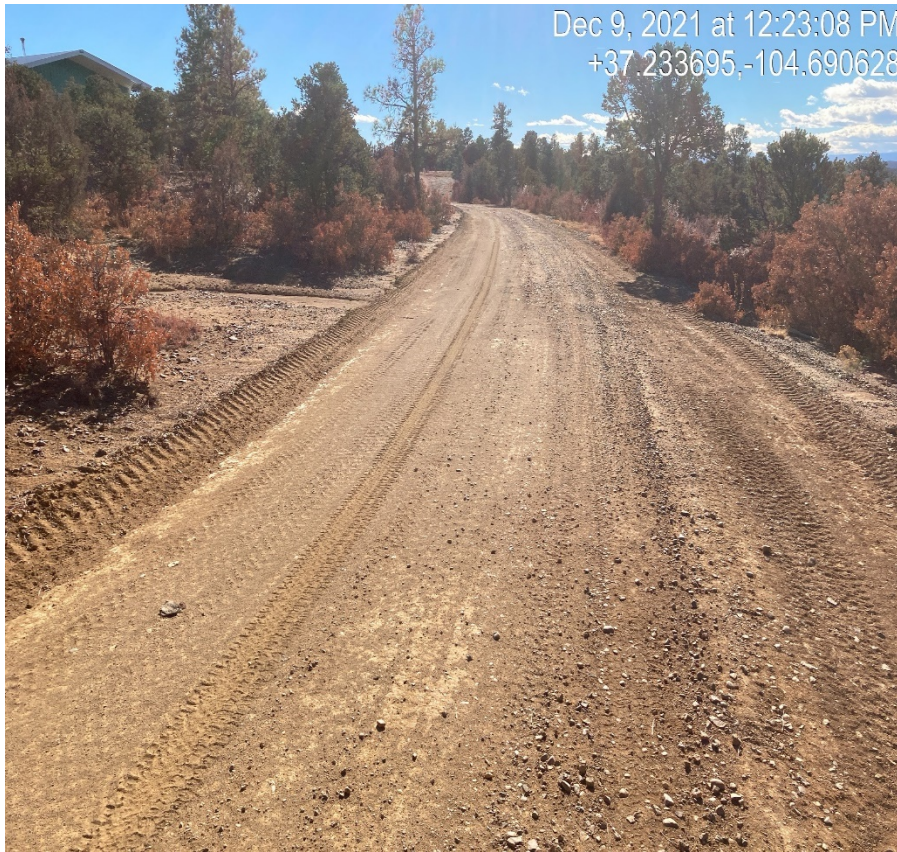
Photo 7. Facing south along the access road. The road was graded however there is insufficient stabilization.
