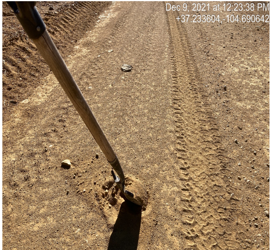
Photo 8. The shovel placed in the road surface shows loose soils and lack of stabilization.
