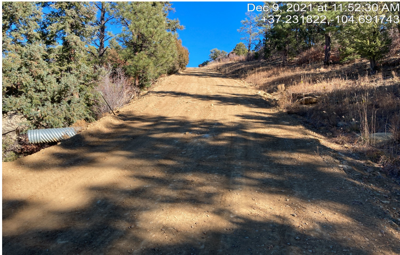
Photo 4. Facing northeast along the steep road. The road was graded however loose soils are susceptible to erosion.
