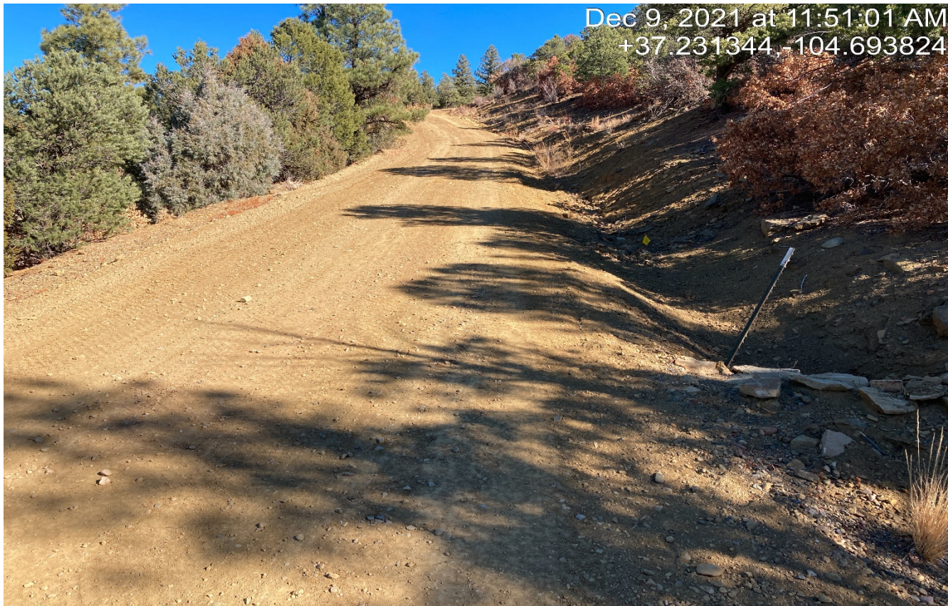
Photo 3. Facing northeast along the steep road. The road was graded however loose soils are susceptible to erosion.
