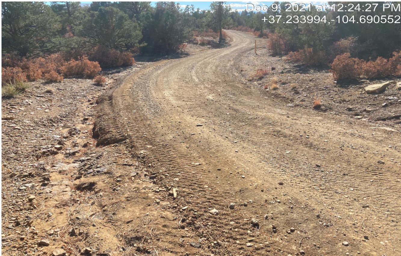
Photo 9. Facing south along the access road. The road was graded however there is insufficient stabilization.
