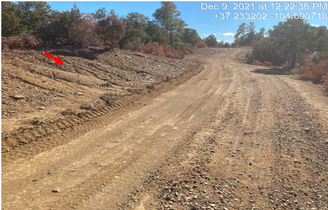
Photo 6. Facing south along the access road. The red arrow shows where erosion is directing sediment onto the road. The side of the road needs to be seeded and stabilized. The road needs to be crowned and stabilized in this area.
