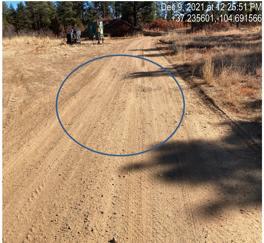
Photo 11. The access road was bladed however the area of water pooling circled has not been stabilized and repaired. This area of the road should be crowned to divert water from the road.
