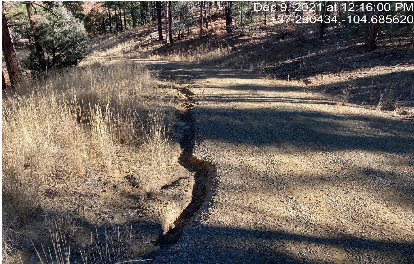
Photo 3. Stormwater is not properly diverted causing erosion of the road.
