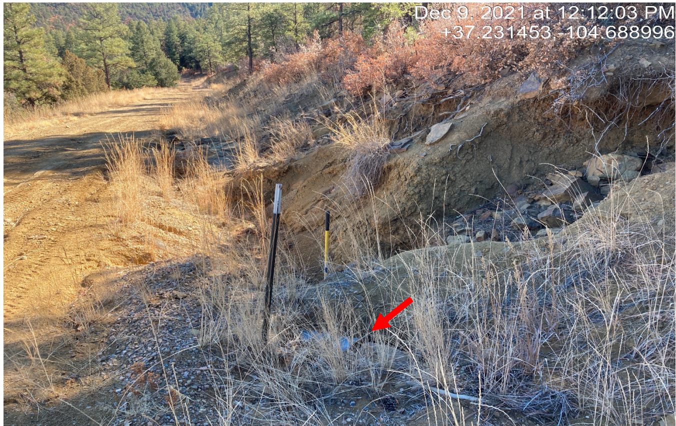
Photo 1. Facing southeast along the access road. There is an erosion gully along the road side. The culvert at red arrow is filled in with sediment and the erosion gully was measured to be 4.5 ft. deep. Previous corrective action was not performed.
