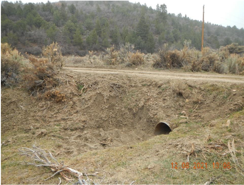
Culvert cleaned out
