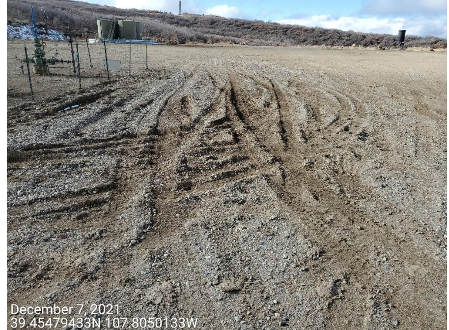
Photo 2: Photos examples showing control measures to stabilize the production area, mitigate tracking, degradation and sediment transport remains inadequate on the Location.
