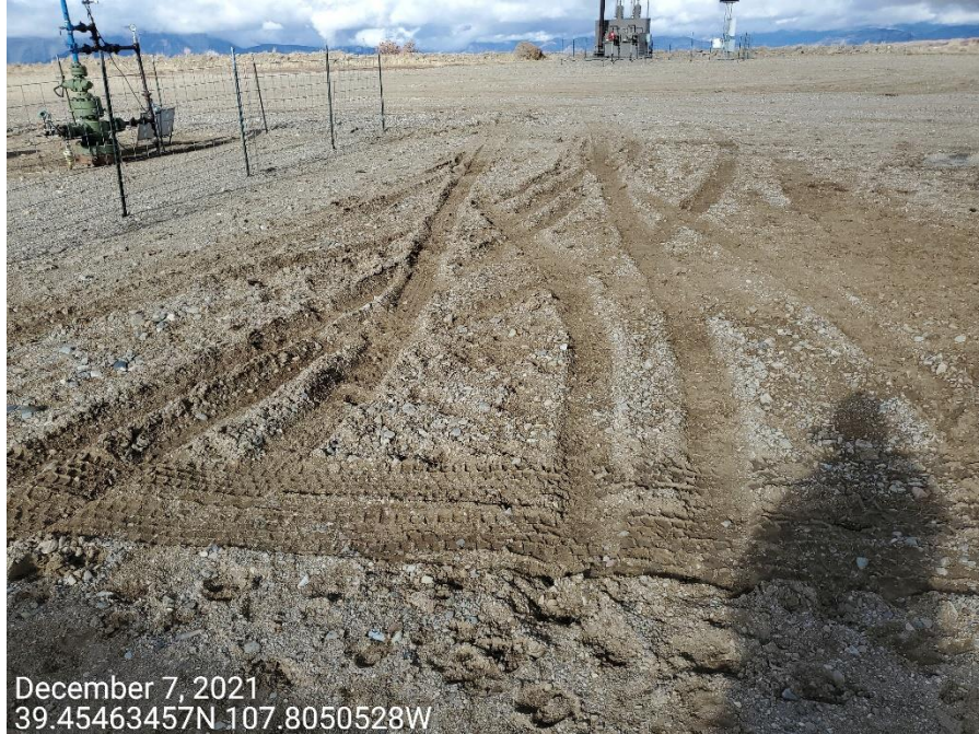
Photo 2: Photos examples showing control measures to stabilize the production area, mitigate tracking, degradation and sediment transport remains inadequate on the Location.
