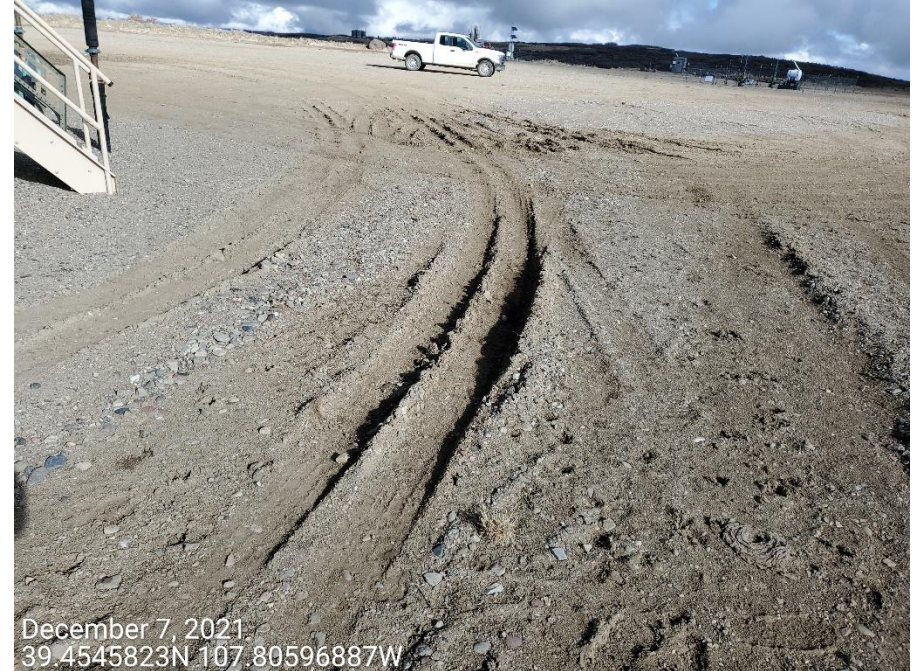
Photo 1: Photos examples showing control measures to stabilize the production area, mitigate tracking, degradation and sediment transport remains inadequate on the Location. .
