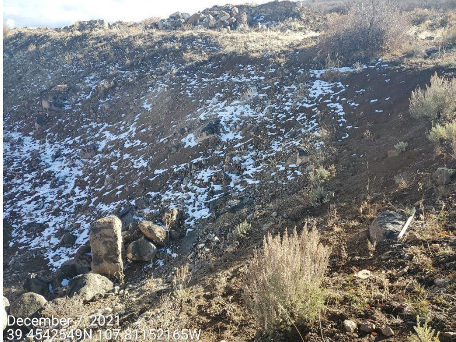
Photo 2: Photos examples showing control measures to protect and stabilize the cut slopes of the Location remain missing or insufficient.
