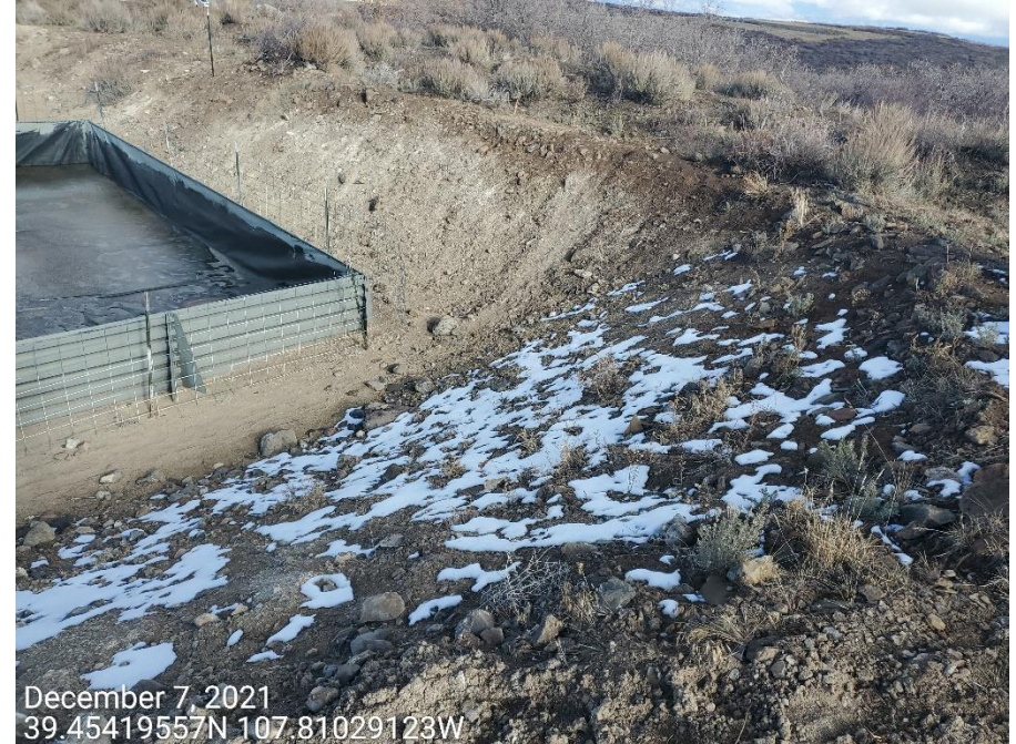
Photo 2: Photos examples showing control measures to protect and stabilize the cut slopes of the Location remain missing or insufficient.
