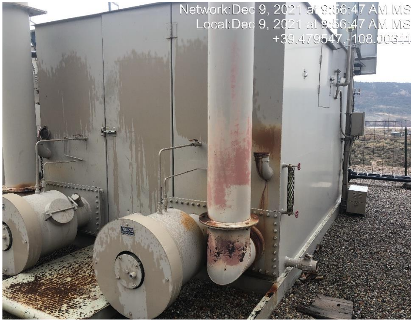
Photo #5373 Storage tanks no labeled.
