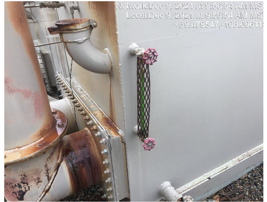
Photo #5374 Sight glass indicates the storage tank is full of an unknown fluid.
