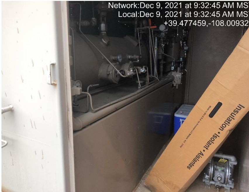
Photo #5369 Storage tank located under horizontal separator.
