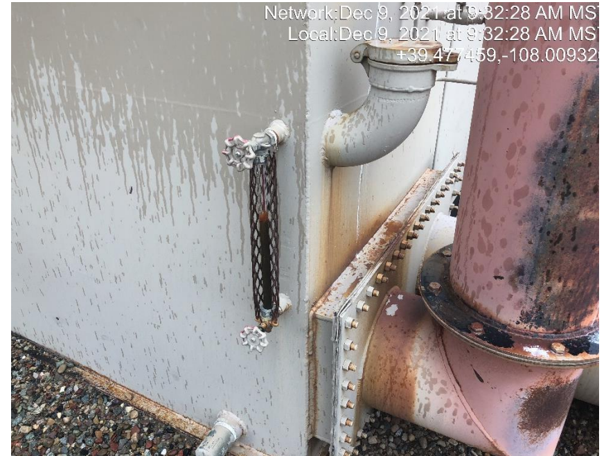
Photo #5368 Sight glass indicates the storage tank is full of an unknown fluid.
