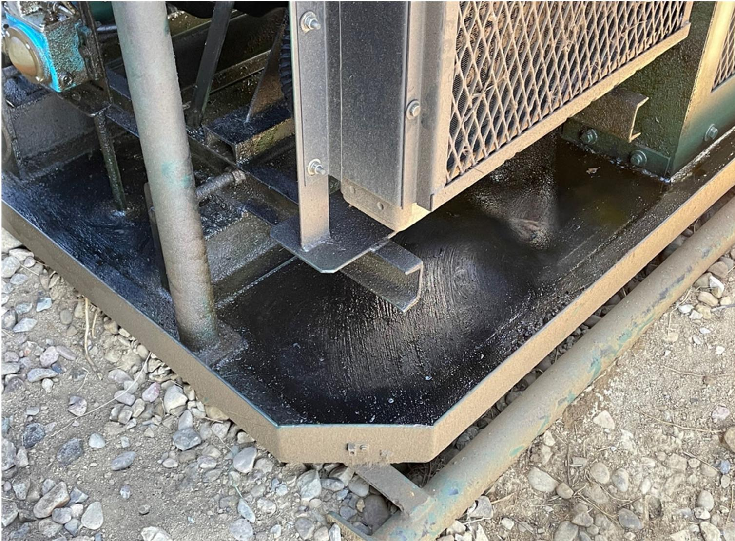
THE FLUID ACCUMULATION THAT WAS FOUND INSIDE OF THE CONTAINMENT SKID OF THE LIQUID RING COMPRESSOR WAS REMOVED.
