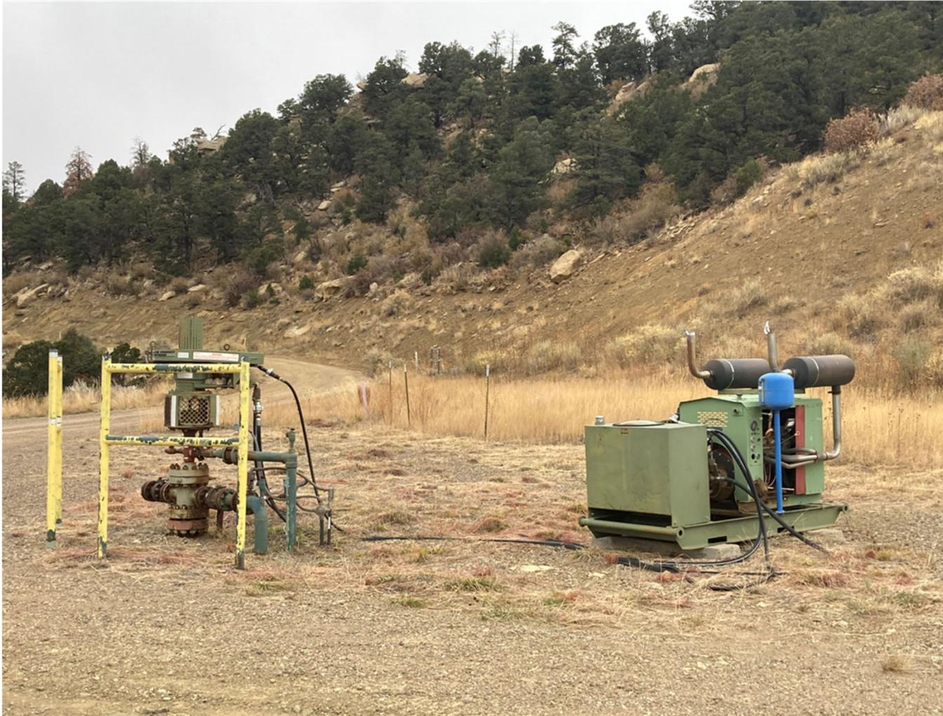
THE VEGETATION THAT HAD ESTABLISHED NEAR THE WELL HEAD WAS CUT BACK AT LEAST 25 FEET FROM THE WELL FOR FIRE PROTECTION.
