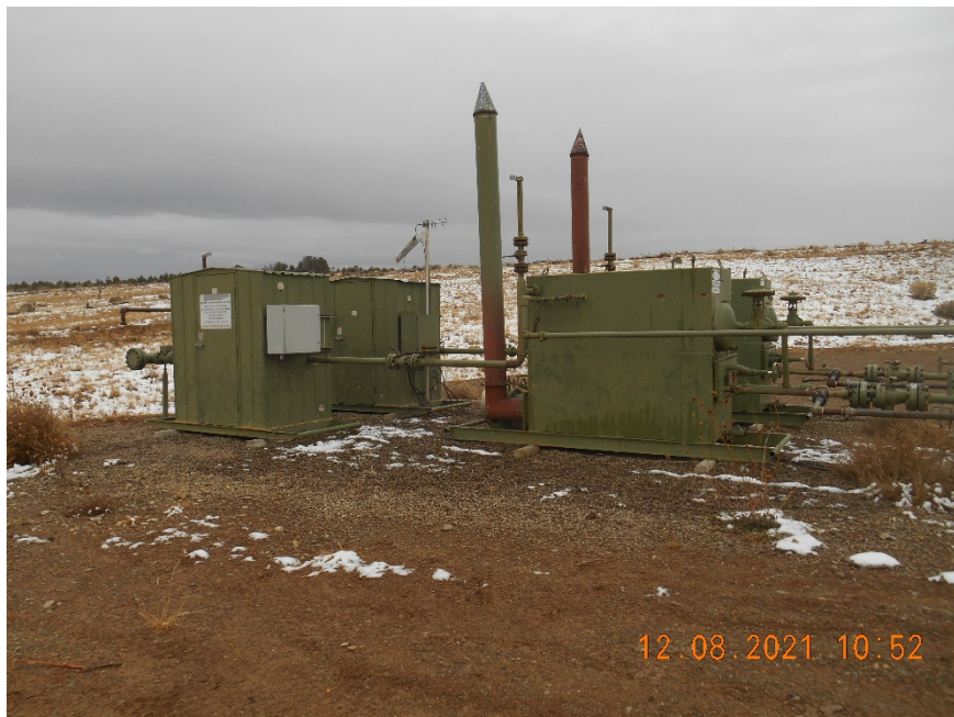
Separators and Meter housings with signs
