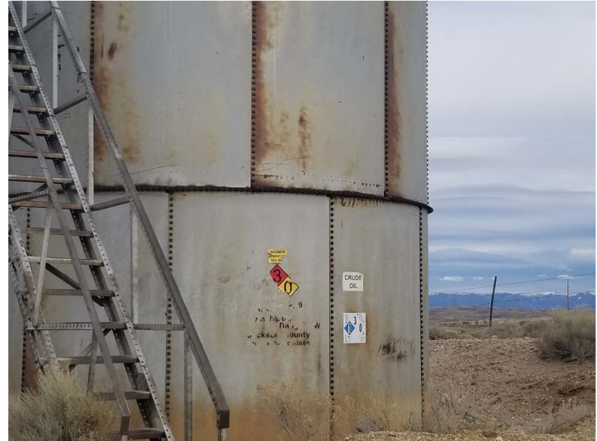
Photo 2. Tank labels faded and peeling.
