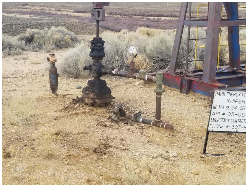
Photo 3. Stained soil at wellhead.
