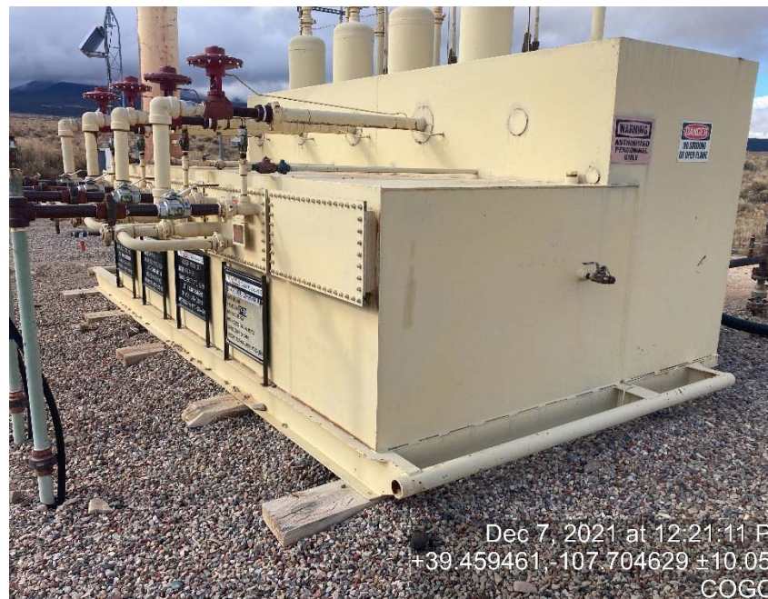
Storage tank lacking label
