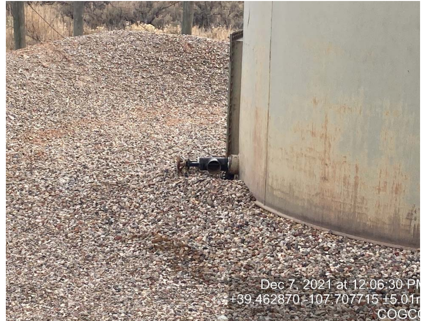
Load line missing bull plug/cap
