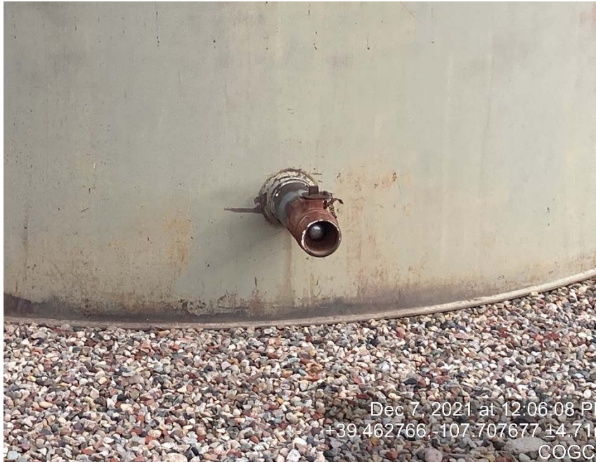
Load line missing bull plug/cap
